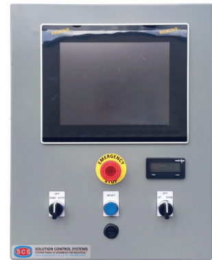
Local Control Panels
